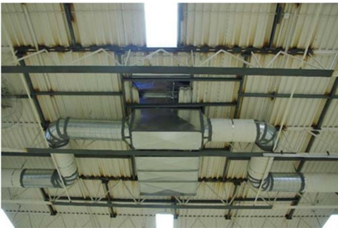
The engineering analysis and new drawings determined that a significant amount of steel was needing to be welded into place to reinforce the existing gym roof before the HVAC unit could be hoisted up and installed. This work and the spray painting to follow took place in late August.
